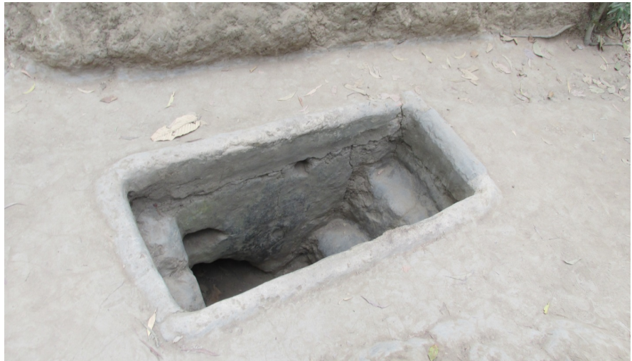
Figure 6. Tunnels were constructed in Old Alluvium lateritic soils where weathered iron oxides made the soils hard like concrete. The soil lining of the tunnel and steps which led up from the tunnels to the entrance were so resilient it was hard for the enemy to destroy the tunnels. This tunnel entrance was preserved as part of the Vietnam War memorial park.
